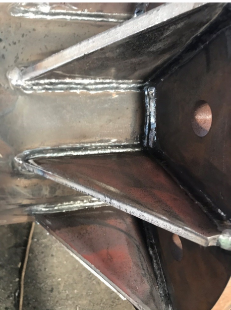
Slipway; Winch Base - Forming & Finish
